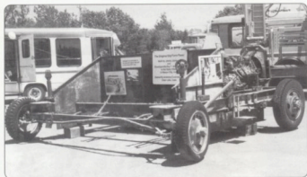
Figure 3: Although it looks nothing like today's slipform pavers, this was the first such machine for road applications. The Iowa Highway Commission's "Johnson paver" is being exhibited by Andrews Concrete of Clear Lake, Iowa, at an unknown venue. Archival photo reprinted from Surface Transportation magazine (3rd Quarter 2006), © 2006, American Concrete Pavement Association, Skokie, Illinois
