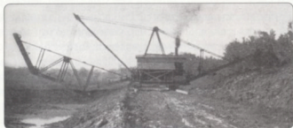
Figure 7: The Swiss Army knife of a machine is the Austin Templet Levee Builder, an indirect ancestor of the machines that first used slipform technology. Image from Excavation Machinery Methods and Costs , Allen Boyer McDaniel S. B., 1919
