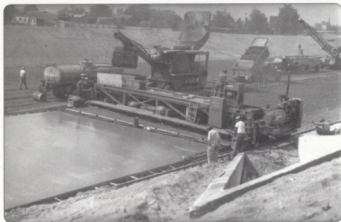
Figure 6: Set up for invert paving, A. Teichert & Son's Guntert & Zimmerman canal paver lays a 24-foot slab in the bottom of the Los Angeles River Flood channel during highway paving simulations in 1956. Photograph courtesy of Guntert & Zimmerman, Inc.
