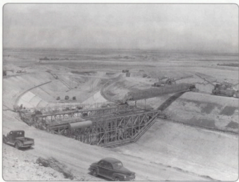
Figure 2: The world's first slipform paver was similar in design to this Guntert & Zimmerman canal paver, working on California's Delta-Mendota Canal in 1947. Photograph courtesy of Guntert & Zimmerman, Inc.
