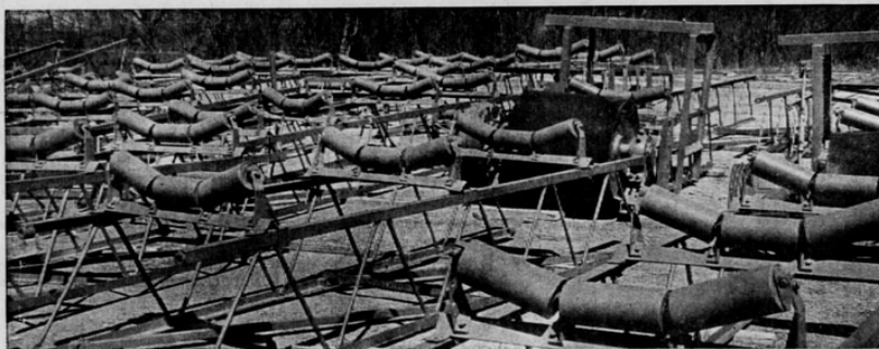
When assembled, these rollers will form a conveyor belt for hauling limestone
